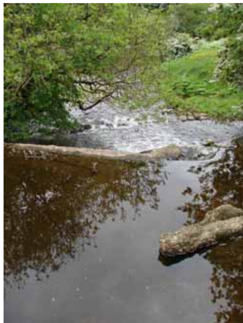
K) Semi-collapsed mill structure
