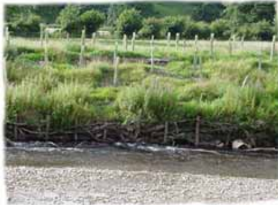
L) Use of willow withies, reprofiling and planting
