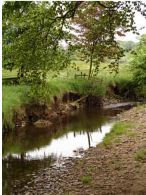
J) Areas of localised erosion
