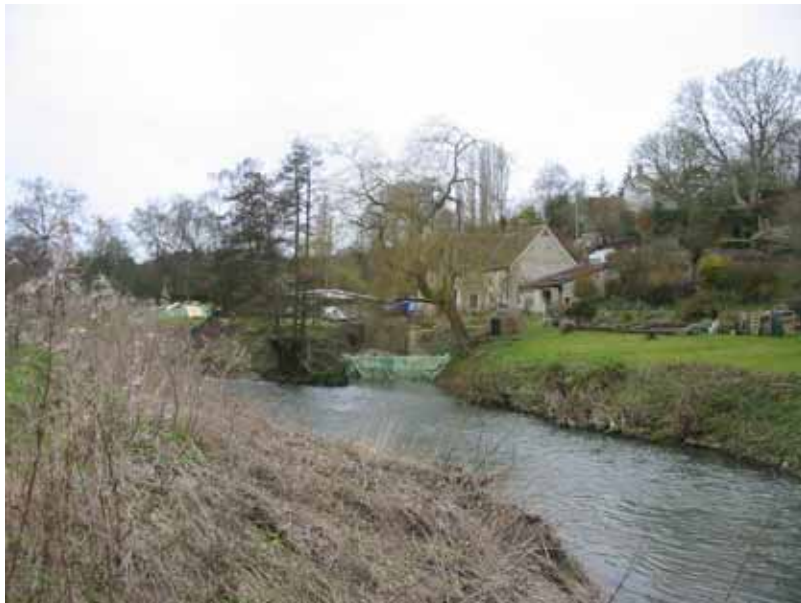
Tellisford Mill showing leat rejoining the main river on the LB
