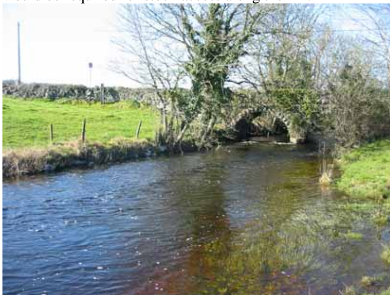
River downstream of bridge
