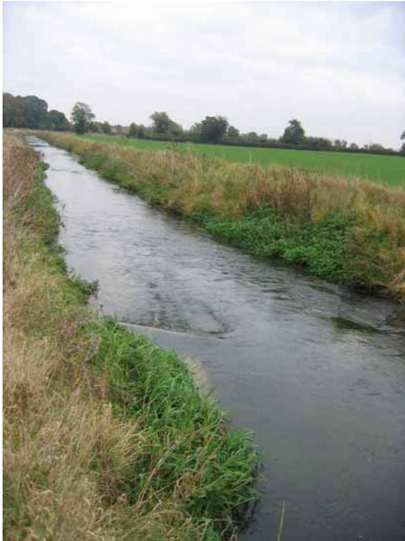
Upstream facing 'v' groynes
