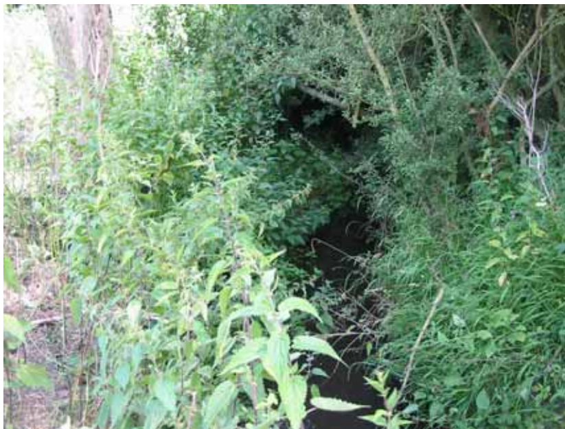
Tunnelled section of the Dodnash Brook
