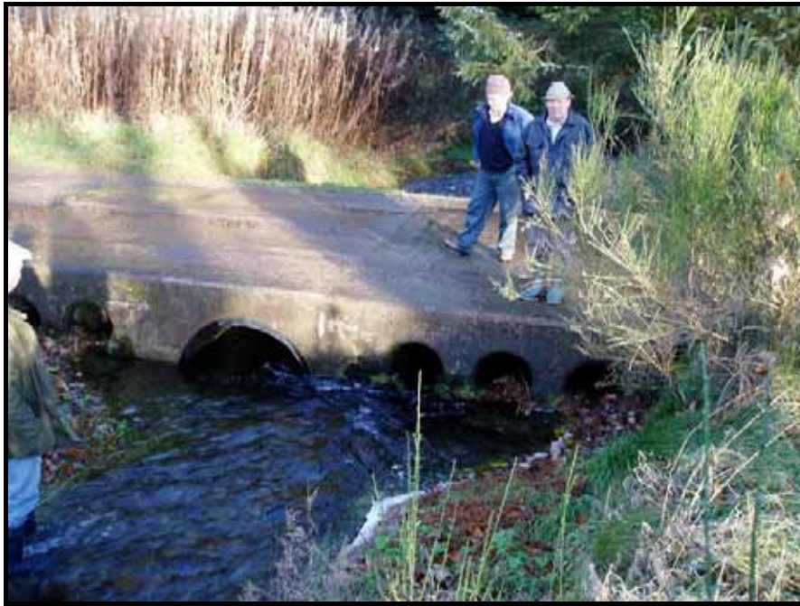
Plate 12: Improved Dutch Bridge in the Lax Burn (Coynachie)
