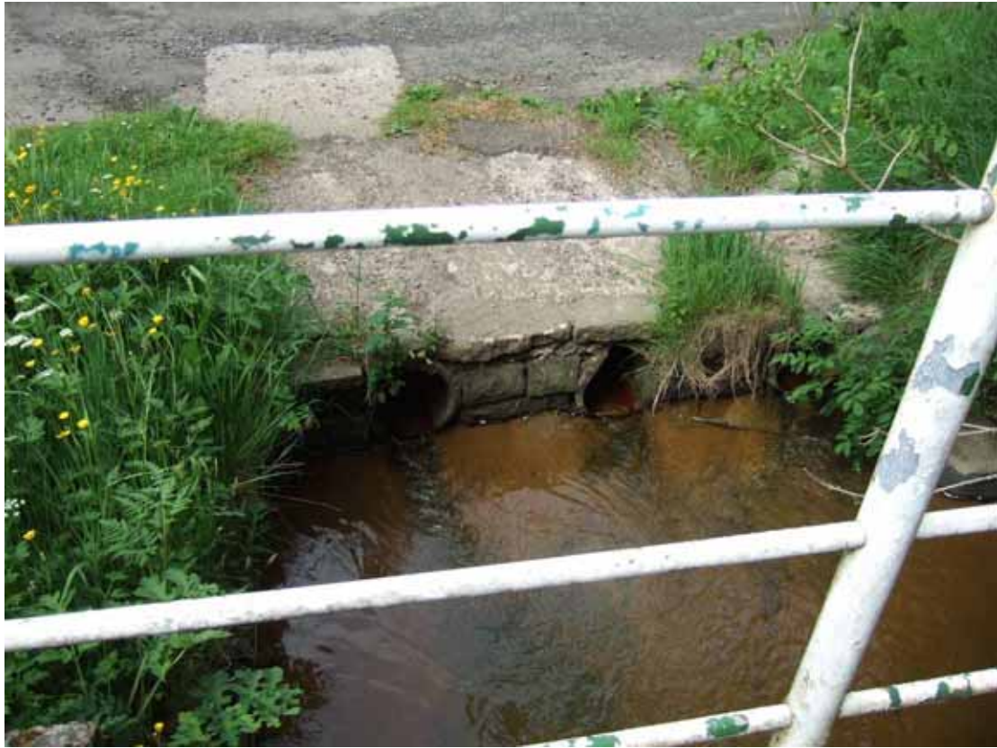
Pipe bridge just upstream of Vindolanda may also require some work.
