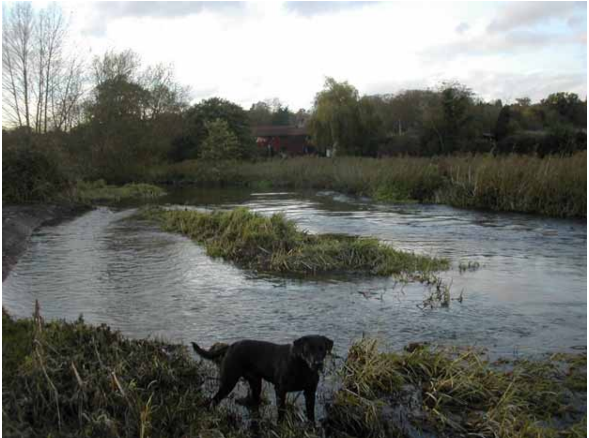
A recently created backwater channel and riffle on the River Wensum cSAC
