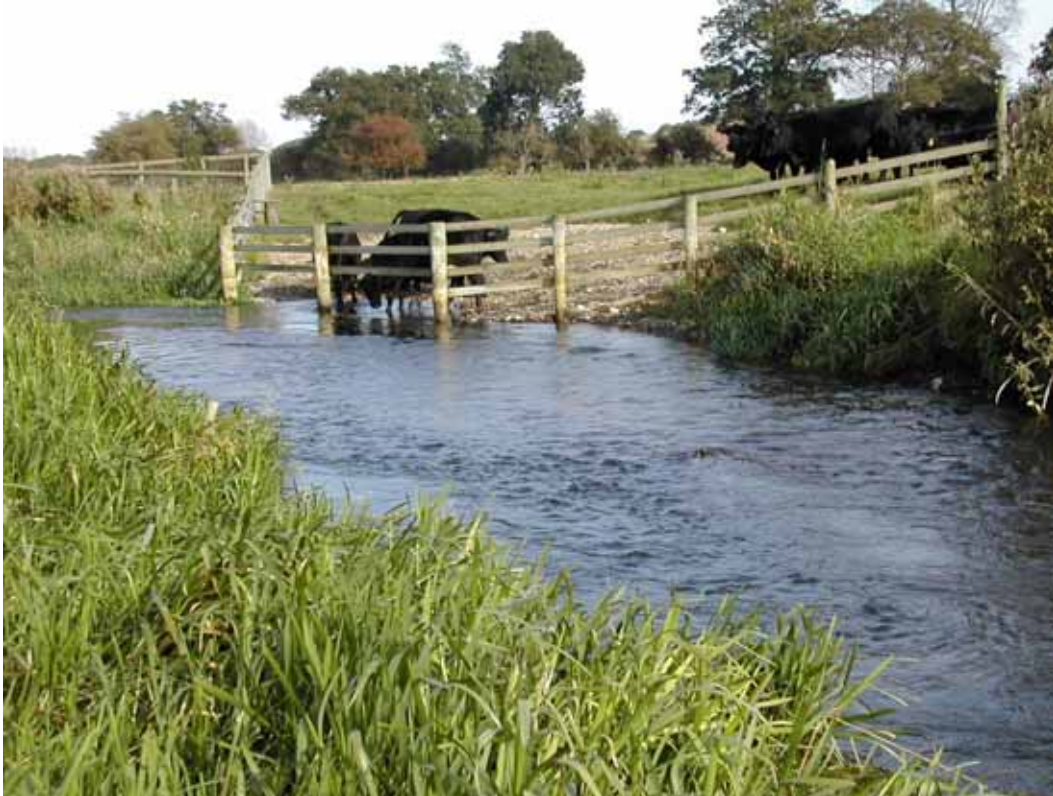
Restoration of cattle drink with fencing to allow safe, clean access for cattle.
