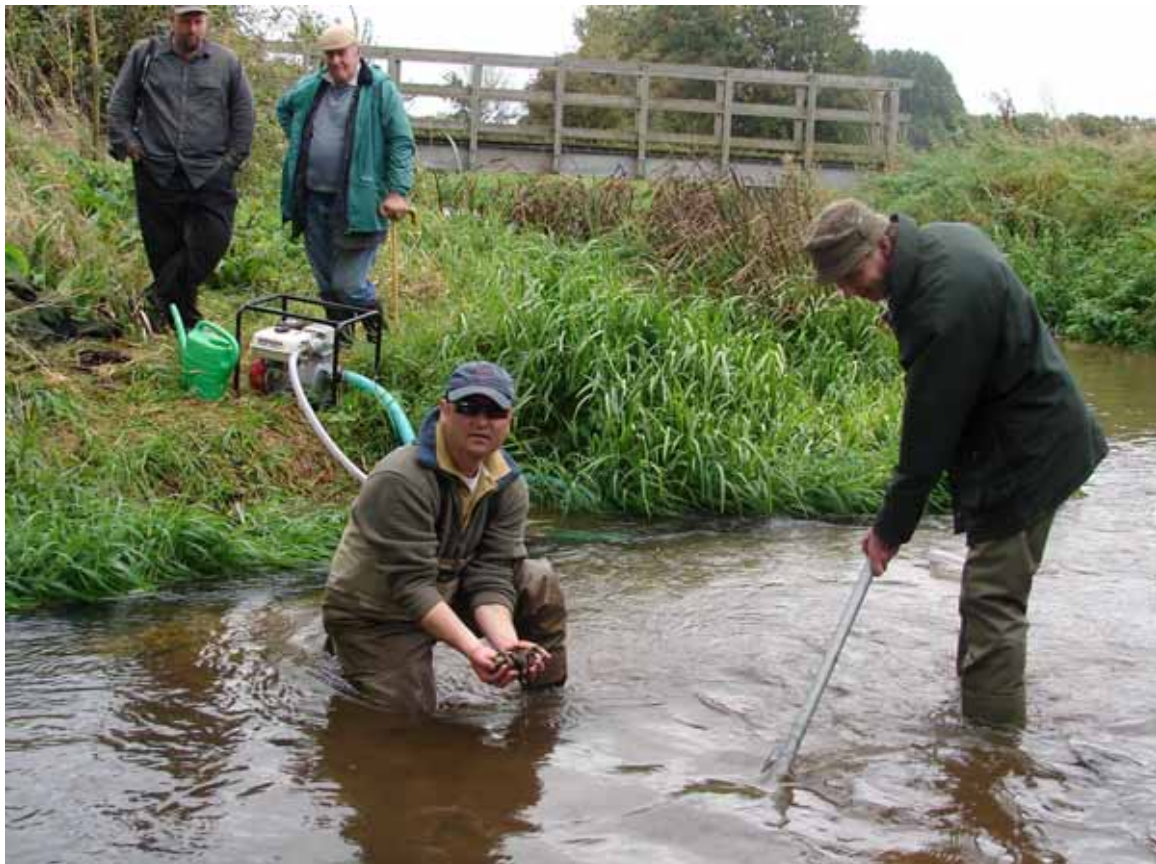
Jetting riffles in September clean prior to trout spawning season
