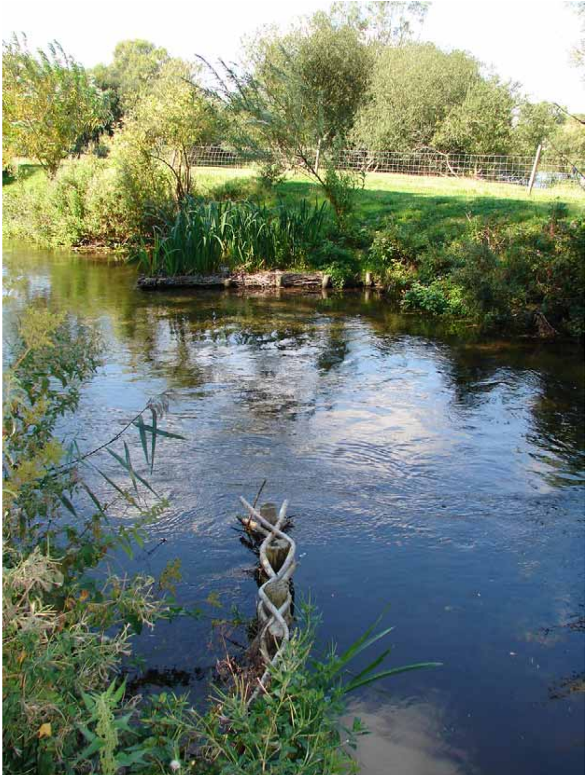
Introduction of single u/s 'natural' deflectors (single, near bank and triangular' far bank) on the Wylde in Wiltshire formed a chicane, sending flow from one bank to another. Note set just above summer water levels.
