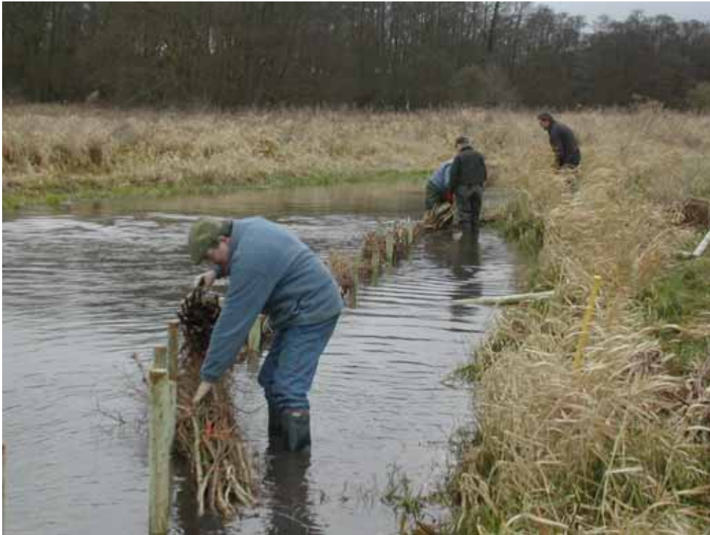
Narrowing Using hazel faggots
