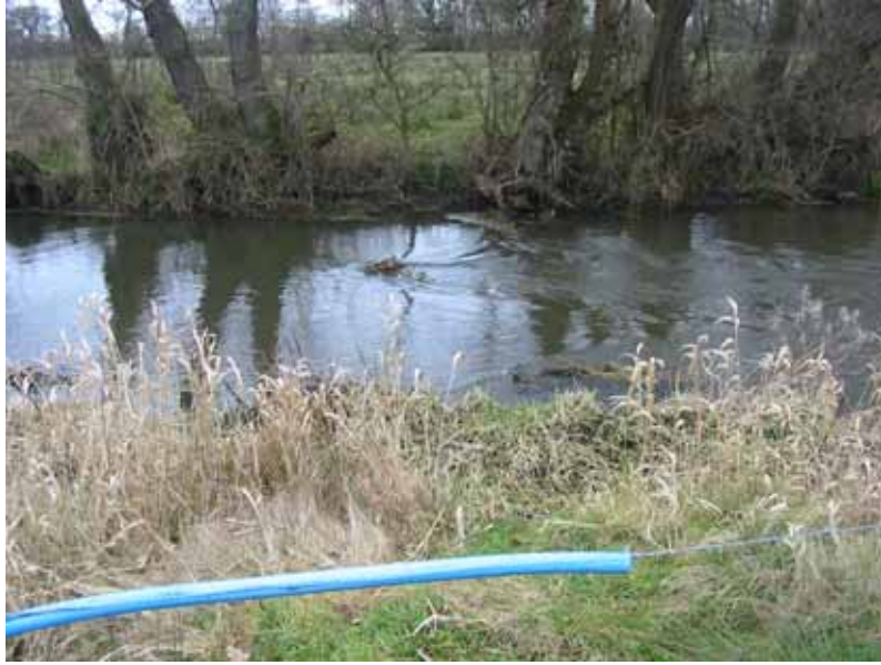
Upstream 'v' groyne
