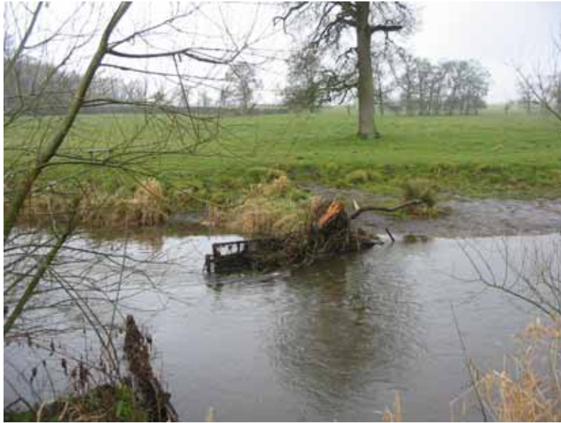
Metal groyne with accumulated LWD on its upstream face
