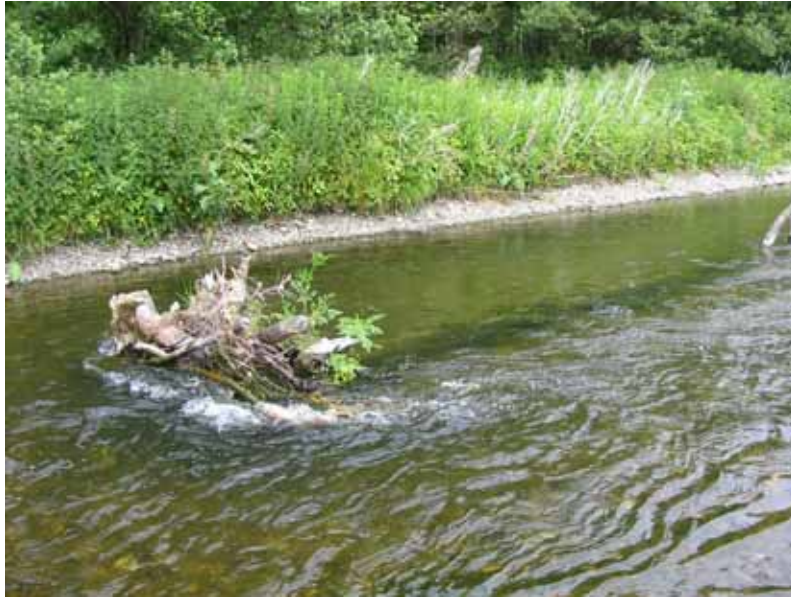
Stabilised tree root system causing localised scour in a river
