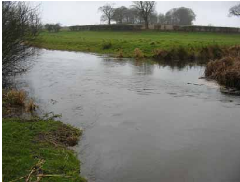
Stone groyne installed by EA fisheries team
