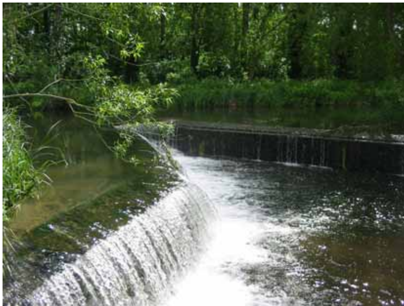
Retaining weir at the downstream limit of the high-level channel
