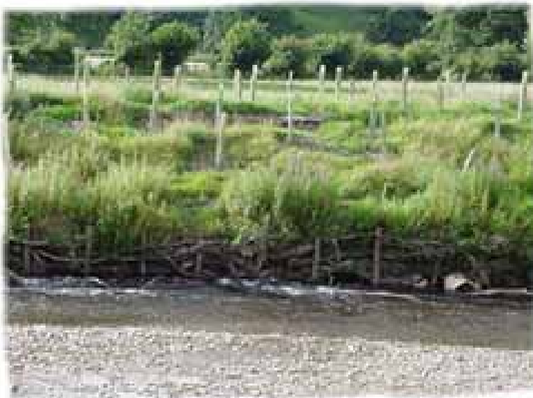
L) Use of willow withies, re-profiling and planting (Copyright Eden Rivers Trust)
