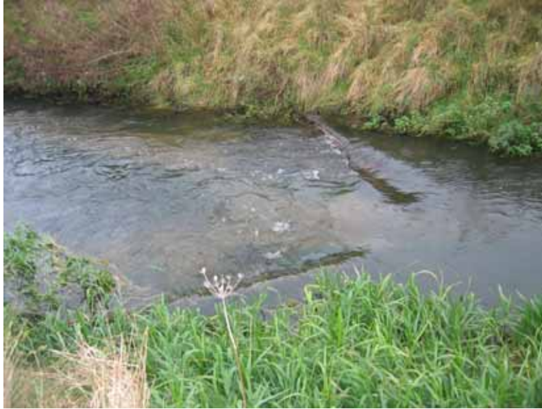
Upstream facing 'v' groyne
