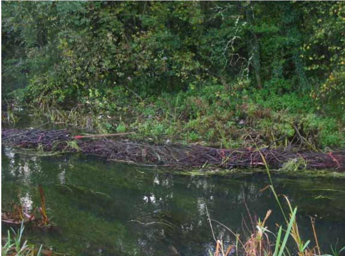
**Faggot bundles installed to narrow stream. Note the growth of emergent vegetation behind the faggot line**
