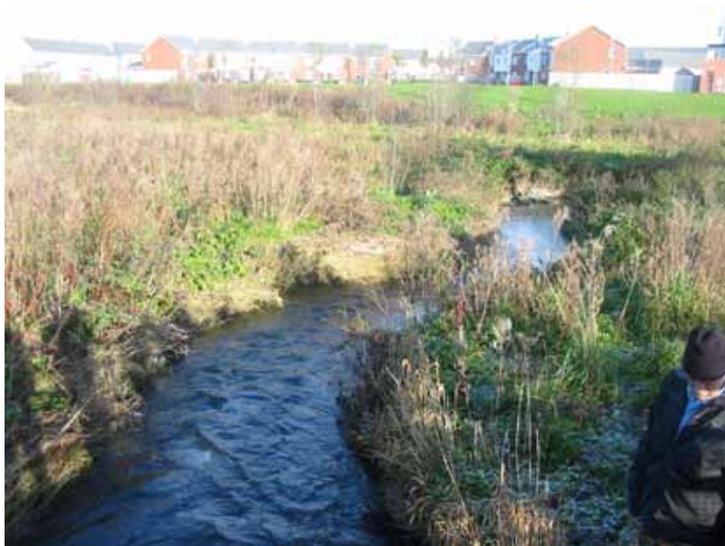
Realigned channel showing steep gradient and high water velocity
