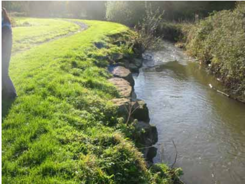
Section of pitched stone revetment
