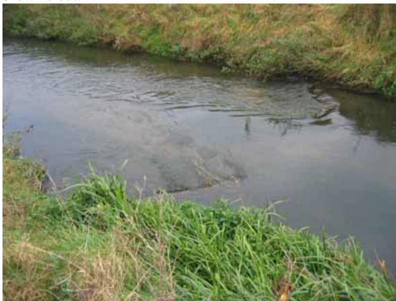
Upstream facing timber groynes showing increased downstream water velocity and scour of spawning gravel
