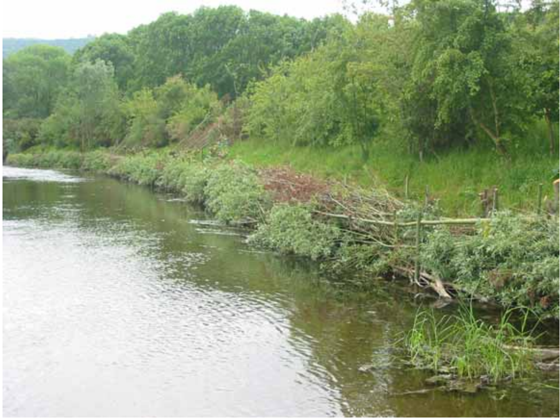
Fenced spiling and tree planting successfully protecting the river bank from excessive erosion
