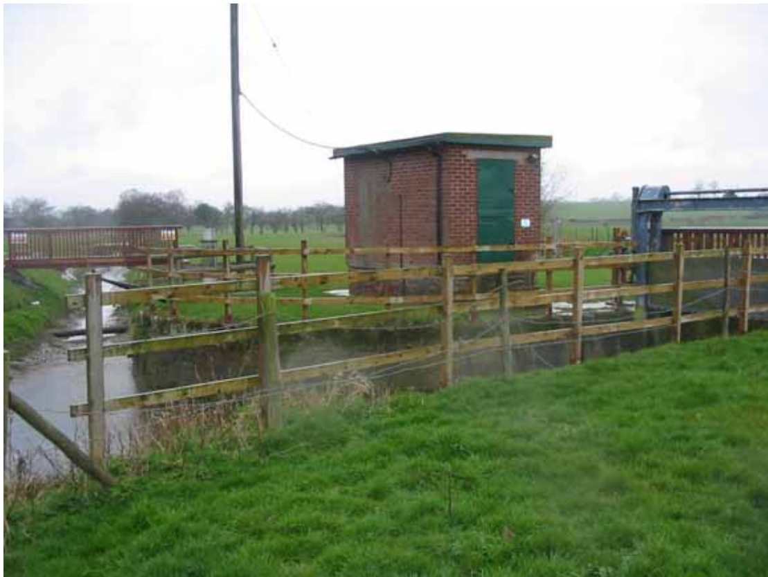
Automated sluice at downstream fishery limit. Note canal feeder to the left of the picture
