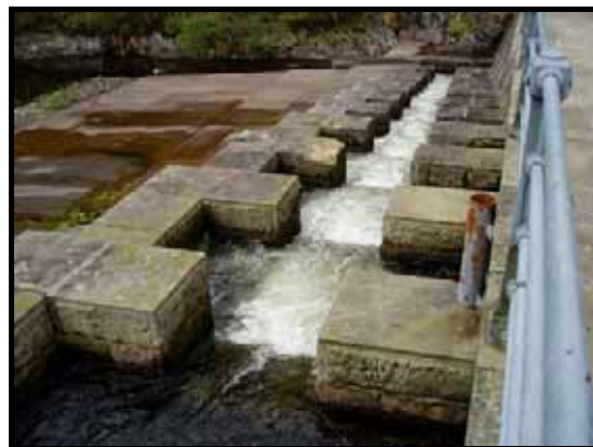
Plate 9: Katrine Dam Fish Ladder
