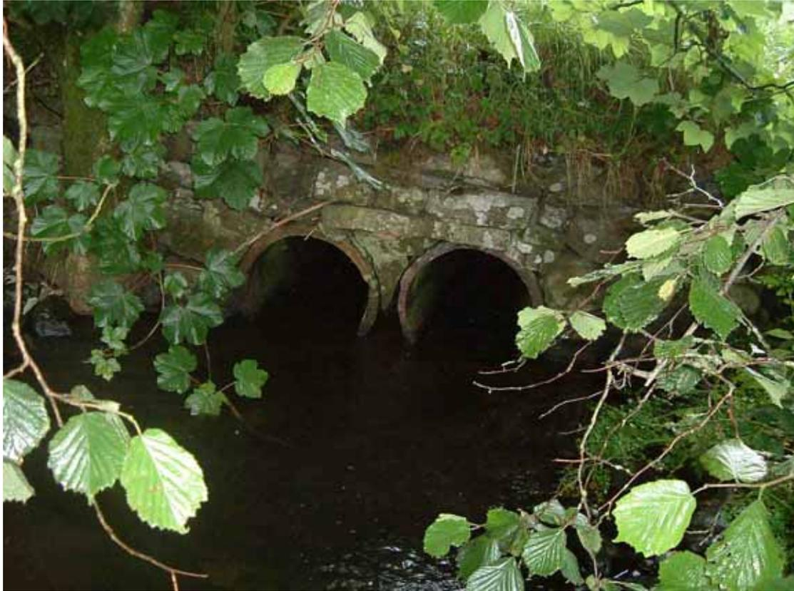
*The culvert is free flowing and passable at these flows but may be a barrier when fish need to migrate.*
