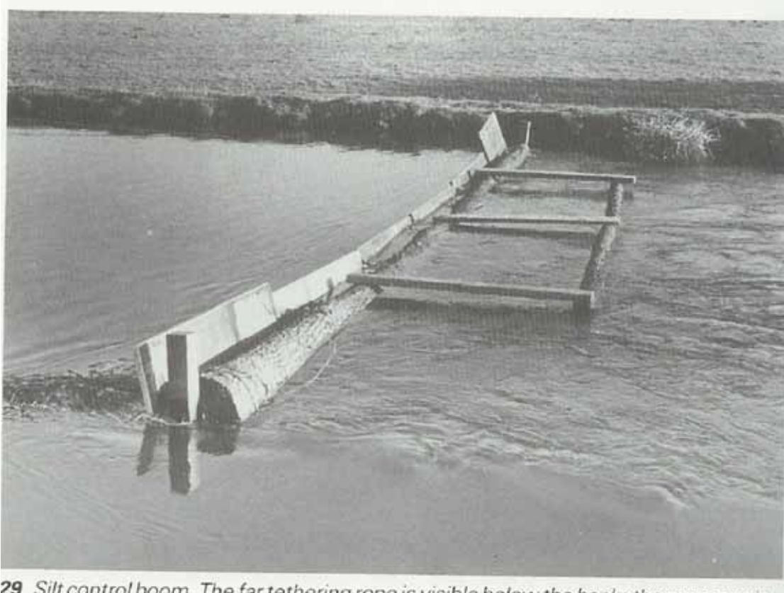
29 Silt control boom. The far tethering rope is visible below the bank; the near rope is
