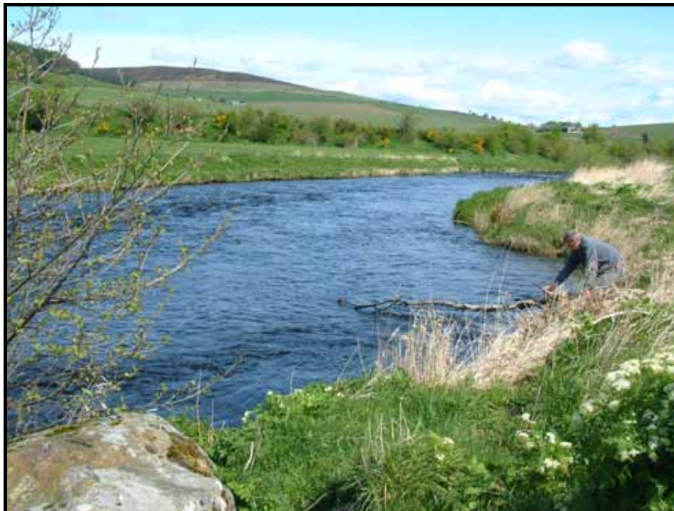
Plate 5: Only very limited bank erosion
