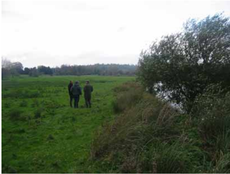
Elevated bund on the RB of the river
