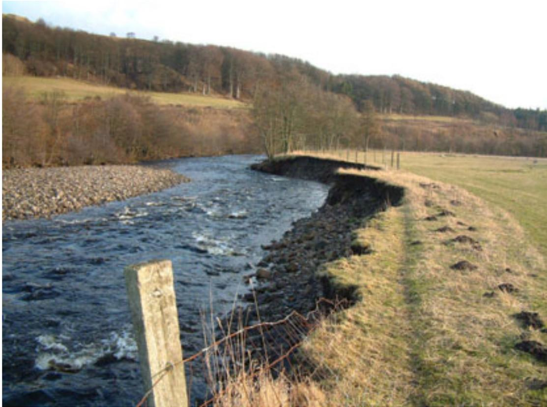
*Accelerated erosion on right bank.*
