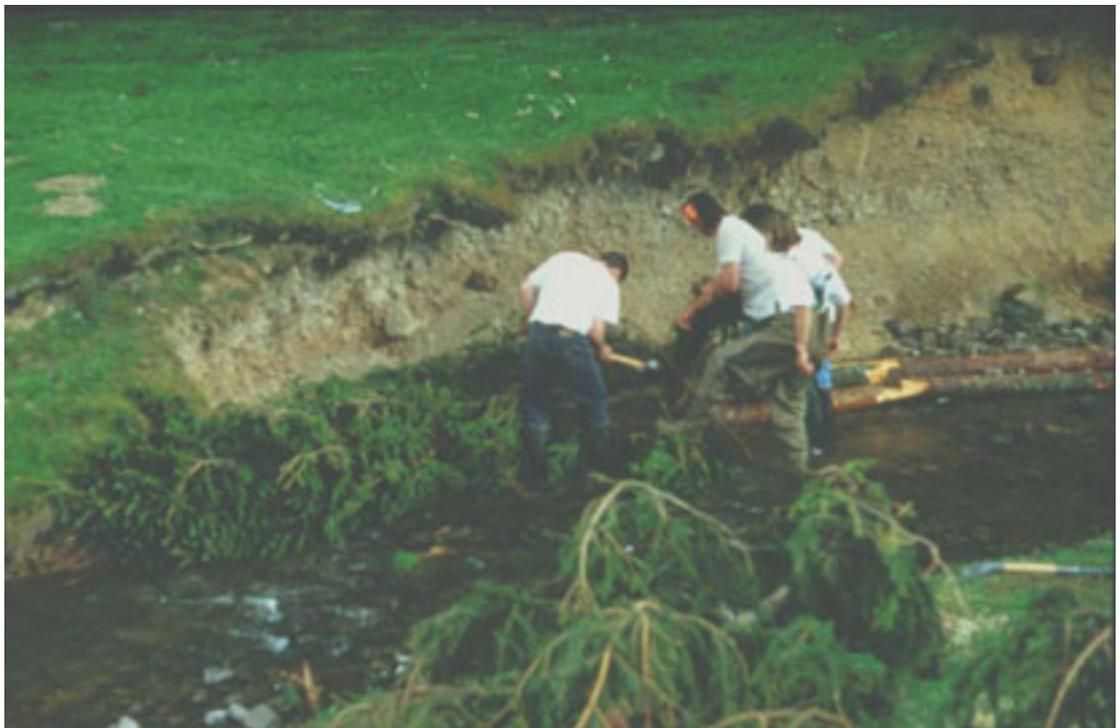
*Larch poles are secured to the riverbank toe using long metal pins. Christmas trees are then nailed to the poles in a downstream facing direction. This method can be replicated using any wood and brush combination, including live willow.*
