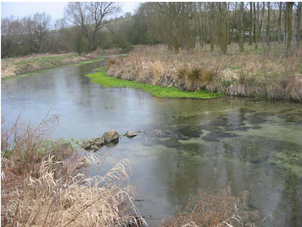
**Overwide channel upstream of bridge, with Sarsen stones introduced to create a low level weir**
