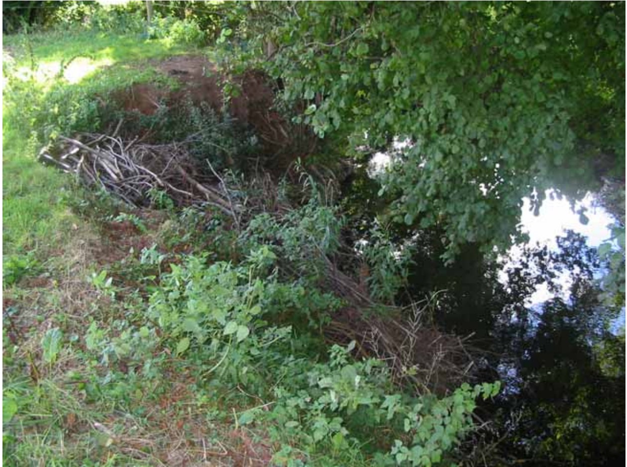
Live willow and deadwood faggot bank protection. Note growing willow cuttings in centre of picture
