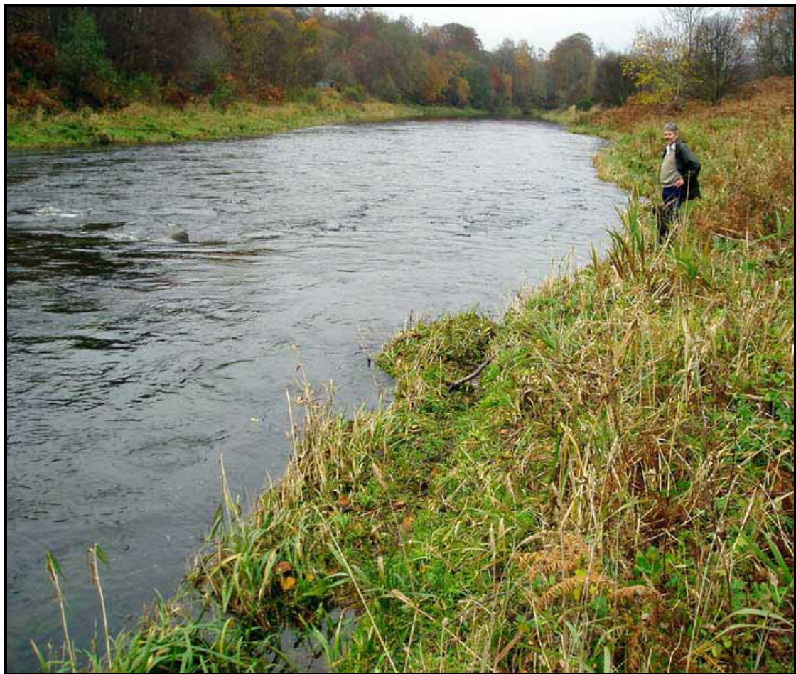
Plate 3. Bank collapse on Garples at the Shark's Fin
