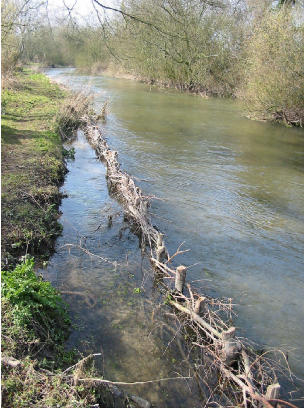
Photo 1: Live willow spiling on RHB of Wylve
