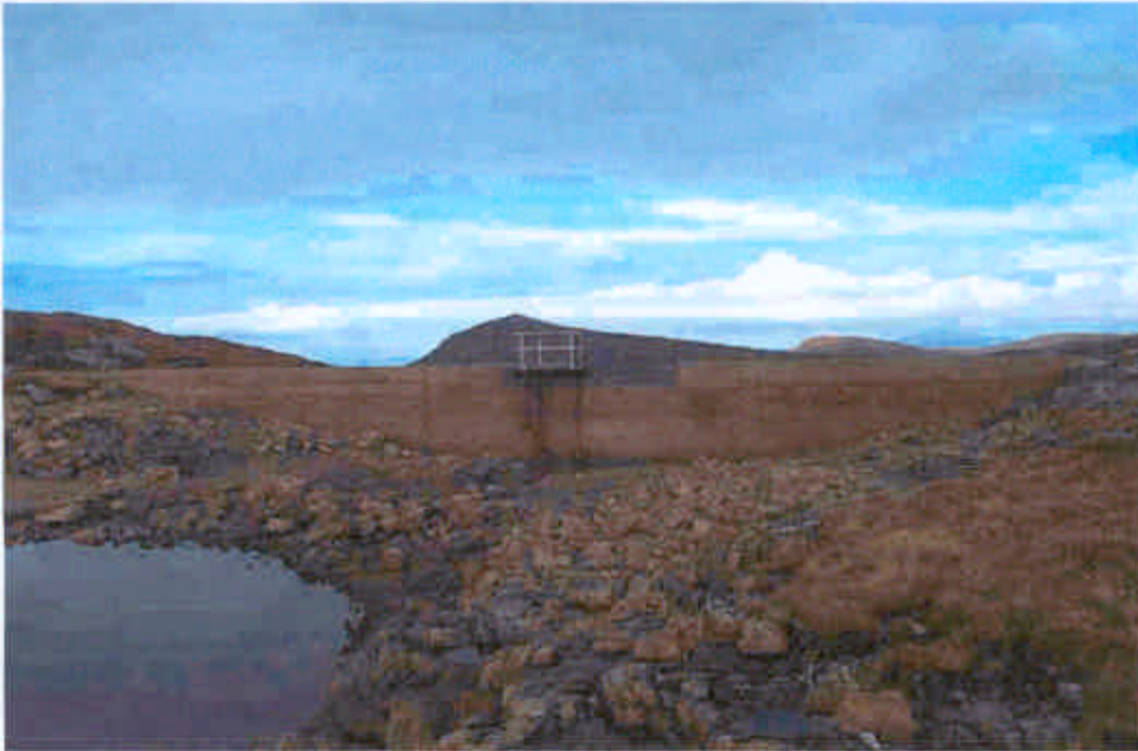
Photograph 1. Dam at the exit of Loch Uisge.
