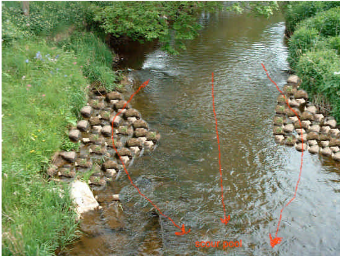
Picture Four – Rock Deflectors
