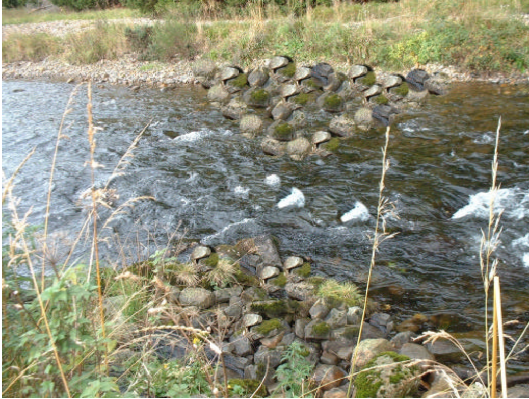
Picture Three: Suggested Rock Constrictor.
