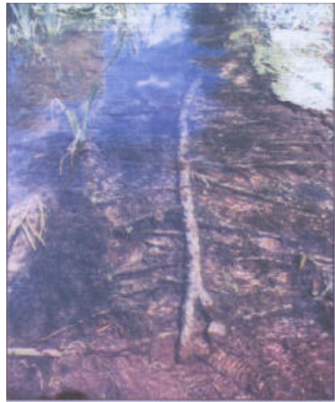
Photo 7. Detail of brushwood structure showing sediment infill and vegetation colonisation
