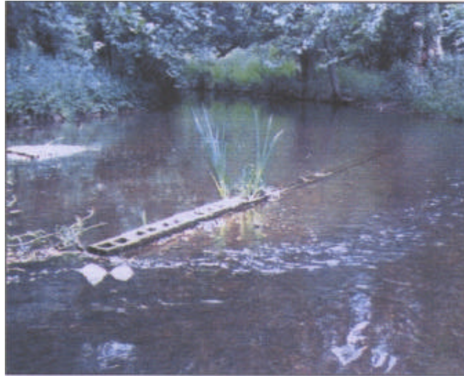
Photo 5. Block installation in Section 4 with ponded area and island to the left.
