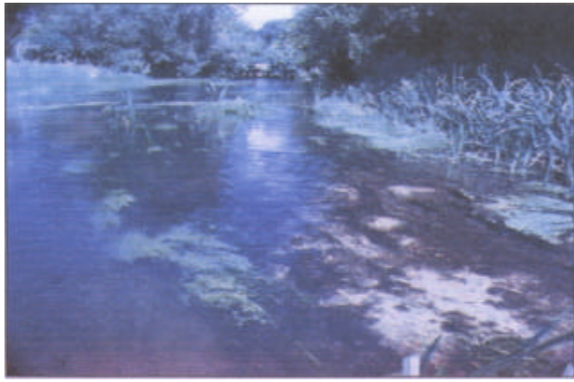
Photo 6. Example of marginal and emergent fringe habitat creation using brushwood mattresses - ideal for swim-up fry- natural sedimentation processes have accreted the brushwood structure during first winter.
