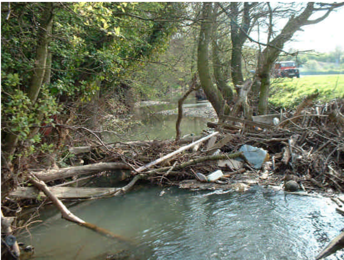
Debris Dam. Pic.1
