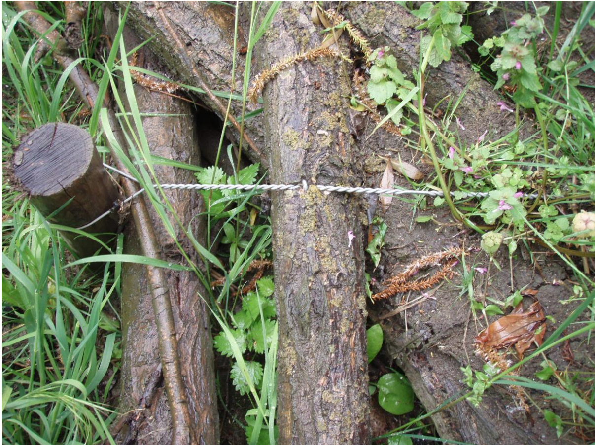
Figure 5 Plain fencing wire and staple method of securing LWS structures to driven posts.
