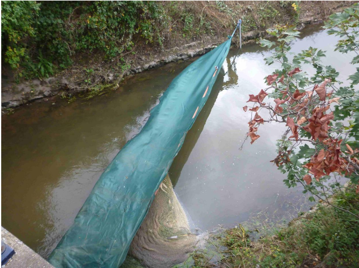
Figure 6 Example of effective Silt control measure – permeable sheeting filled with straw and weighted, stretched across channel between ratchet straps.
