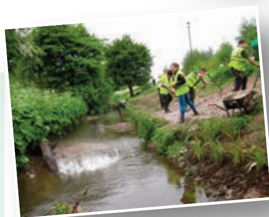
Gravel addition, woody material installation and planting by volunteers in a well-used urban park on the Lyme Brook.
