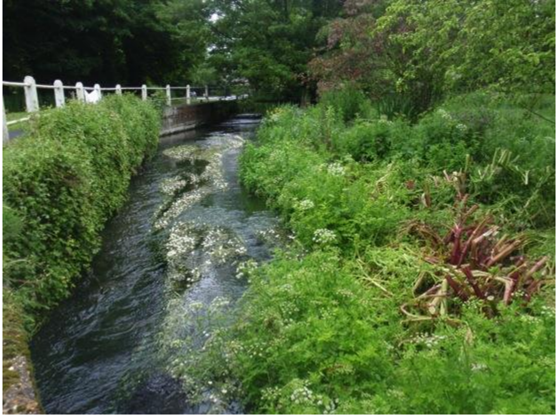
The first 3 Fly event in 2010 raised funds that contributed to this work on the Meon at Meonstoke, where the true left, concrete-lined bank has been softened with a vegetated berm and a weir, just visible in the background, has been notched to ease fish passage.
