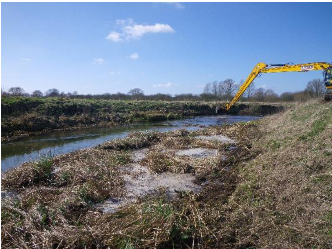
Boggy berm installed with run & pool created on the the tail
