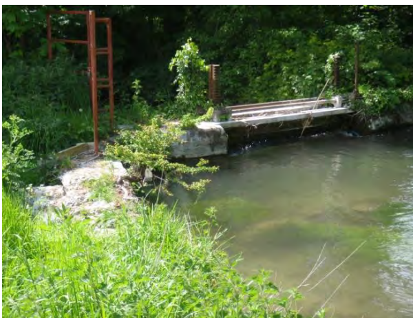
Winchester College structure
