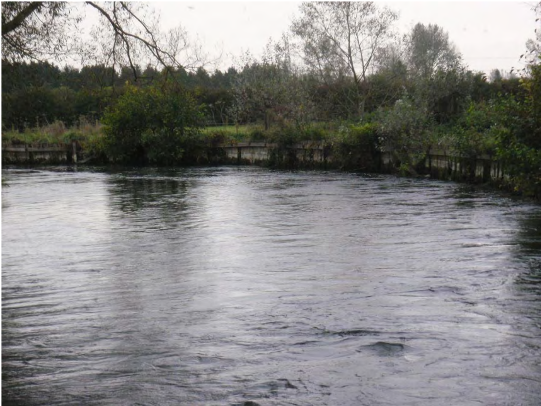
110m of wooden piling true right bank
