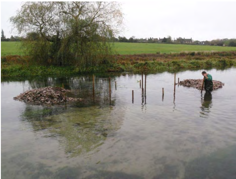
First island being built – notice near bank mobilisation of silt already due to increased velocities.
