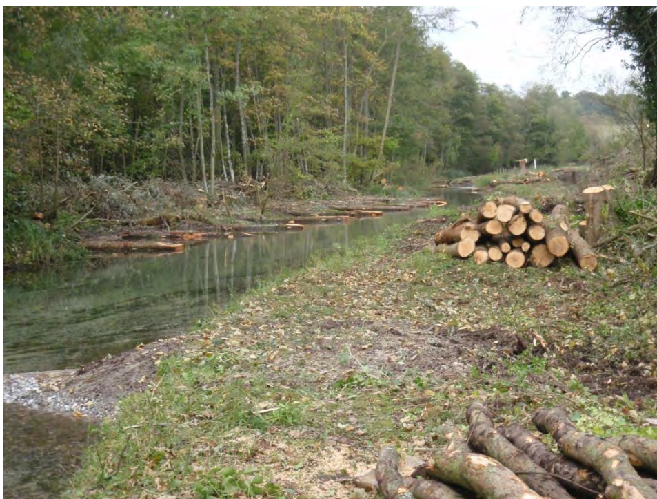
Tufton phase 2 – work in progress
