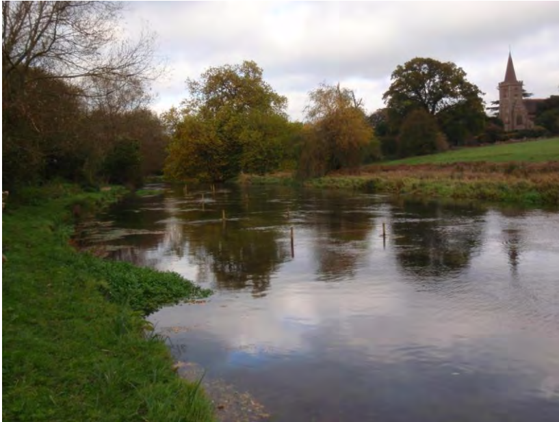
Looking upstream – view of over wide, slow, dredged section with islands staked out.
