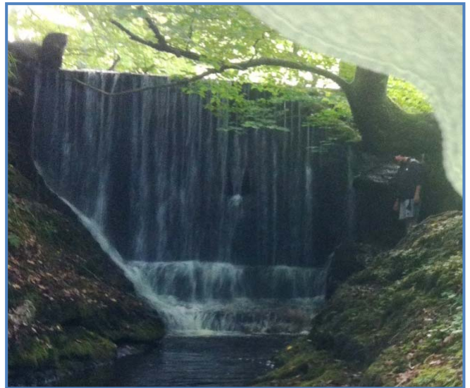
Volunteers from Gardenstown helped survey of the Tore Burn, near Troup Head, and discovered this weir which stops migratory fish accessing the upper half of the Burn. Volunteer, Tom Bean, on the right, shows the scale of the obstacle.
