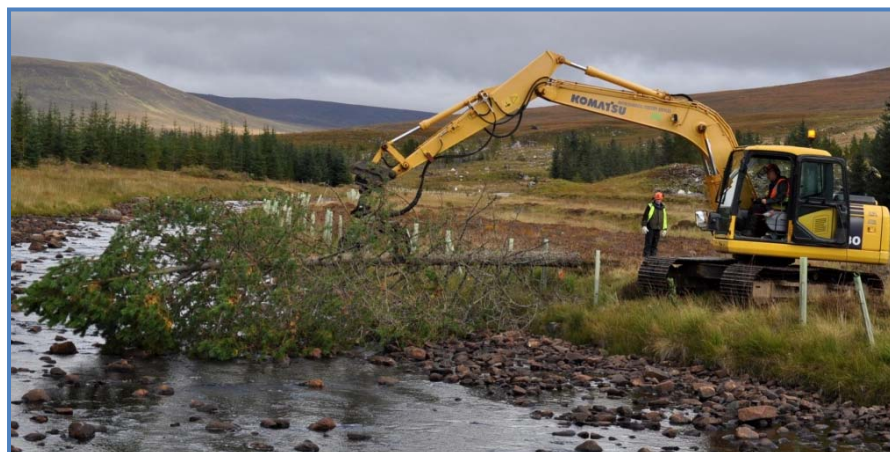
FCS installing LWD into the Strath Rannoch to help improve in stream habitat diversity.
