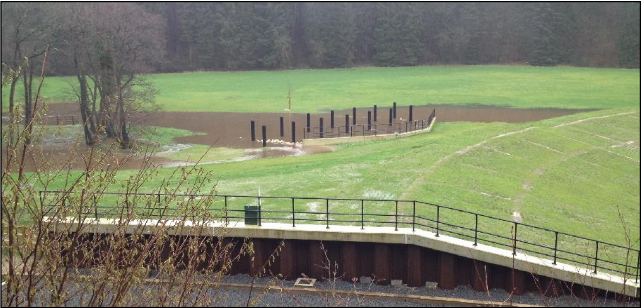
Plate 1 – View of flood storage area at Newtondale during the Boxing Day 2015 flood event.
