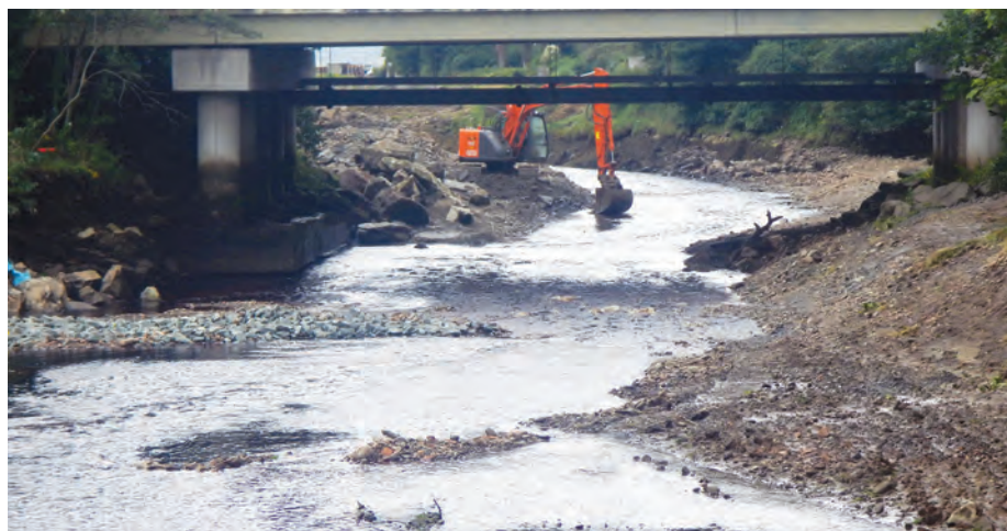
Above: In-channel dredging on the Mill River during the visit. Below: Kayak surveying on the River Pollagh
