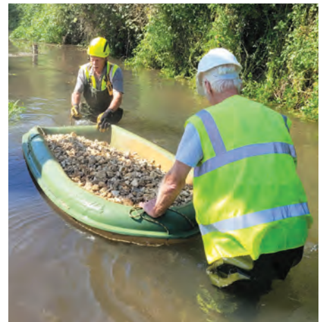
Left: An undredged section of the Lyde. This is what the river should - and will - look like! Above: The boat-as-wheelbarrow technique for moving gravel
