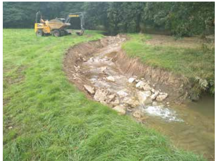
Work on the Brailsford Brook: clockwise from top left, lowered water after a weir removal, exposing many signal crayfish burrows; natural features reappearing though a good flush still needed; a notched weir to improve fish passage; a bypass around a retained weir
