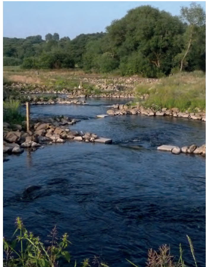
Figure 2. Nature-like bypass channel construction and naturalisation (various viewpoints).
