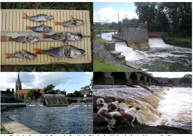
Clockwise from top left: perch sliced in half by hydro blades; hydro turbines on the River Mole in Surrey; salmon leaping over Hexham bridge footings; an artist's impression of Marlow weir with Archimedes screws installed.
