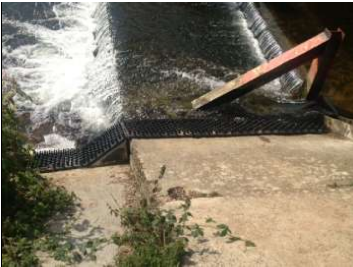
A row of eel tiles installed at Maxey Road
