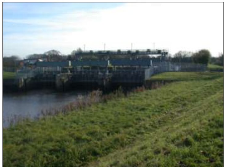
Marsh Road Sluice, Spalding: a major barrier to sea trout passage between the tidal and freshwater Welland.
