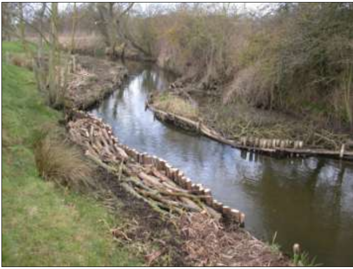
Channel narrowing on the Gwash at Ingthorpe
