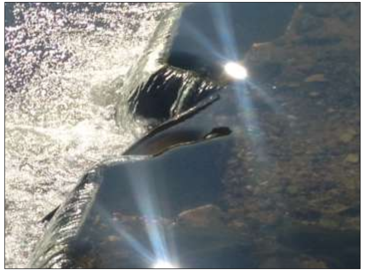
A notch cut in a sheet-piled weir to improve passage
