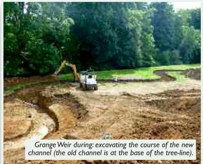
Grange Weir during: excavating the course of the new channel (the old channel is at the base of the tree-line).
