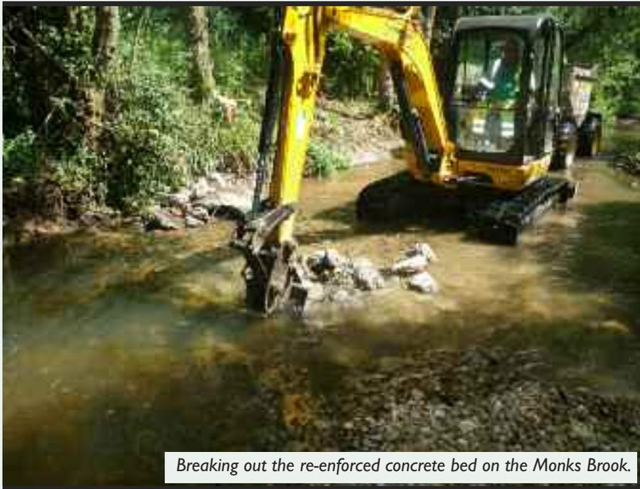
*Breaking out the re-enforced concrete bed on the Monks Brook.*
