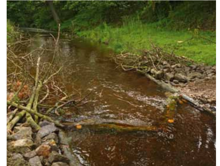
Artificial pinch point generates sufficiently focused flow for a paired ‘upstream-V’ flow deflector to operate. The V deflectors are designed to produce a scour pool in the centre of the river channel (also generating a downstream mound of spawning gravel). Nearby bolt-hole refuges have been provided by brash (loose sticks, branches and vegetation) nailed to the logs used to construct the pinch point and extra submerged cover will be added subsequently.
