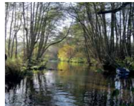
Restoration in progress: Dave Brady from the National Trust and his team winching LWD in place on the Bure, November 2010
