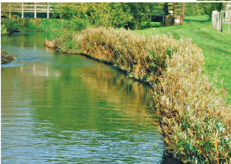
Live willow spiling installed on the outside of a bend
