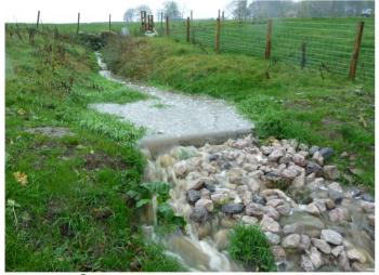
Small ( $\approx 10\text{m}^3$ ) instream detention feature from which soluble reactive phosphorus and nitrate-nitrogen data were collected (Eden)
